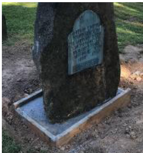
Stage 1, notice the narrow concrete collar around the base of the boulder.
